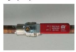
Photo 2a. Ball valve: open position
